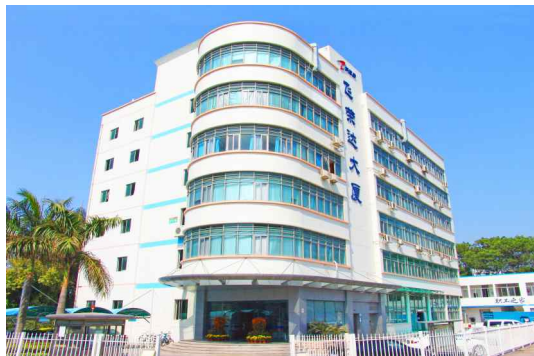
飞荣达大厦 (深圳) / FRD Building (Shenzhen)
